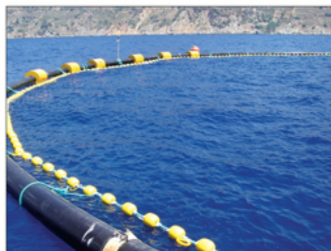
View of installation (Turkey)
